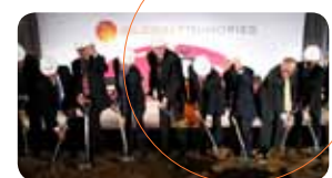
GROUND BREAKING AT FAB 2 – TOGETHER WITH LEADERS FROM FEDERAL, STATE, AND LOCAL GOVERNMENT, GLOBALFOUNDRIES CELEBRATED GROUND-BREAKING FOR THE MOST ADVANCED SEMICONDUCTOR FOUNDRY IN THE WORLD IN JULY 2009.
